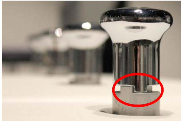
Fig. C-13 Shaft Clamp and Key in Position
